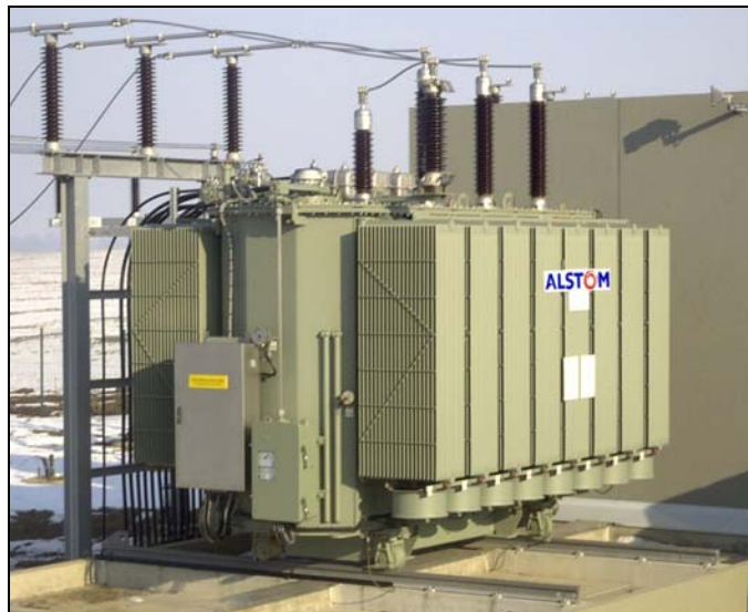
Fig. 5: Hermetically sealed power transformer 80 MVA / 110 kV
